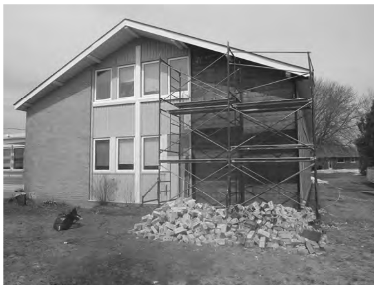
Brick work on front of church renovations April 18, 2014
