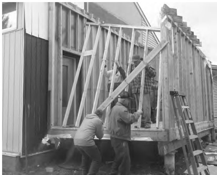
Tearing down the old 'cold storage' at the back of the church May 5, 2014
